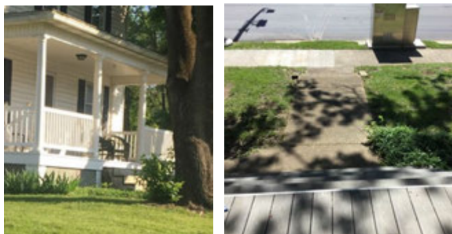
Images of missing railing
