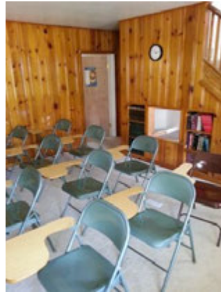
Images of combustible wood wall coverings in classroom and stairway
