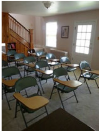
Images of combustible wood wall coverings in classroom and stairway
